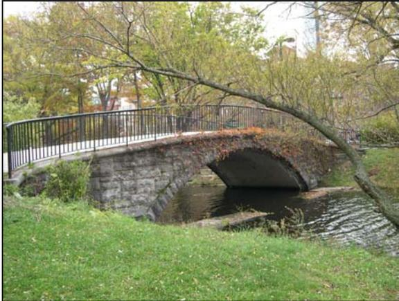
Figure 2.31 – 1930s granite bridge with new railing. (2007).
